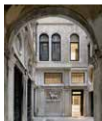
David Chipperfield, Restauration des Vieilles Procuraties
